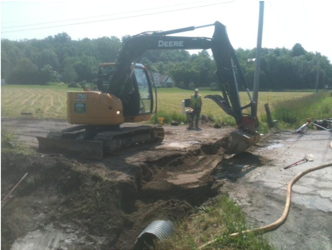
Highway crew replacing a culvert at the intersection of Buck Hill Road West and Rte 116
