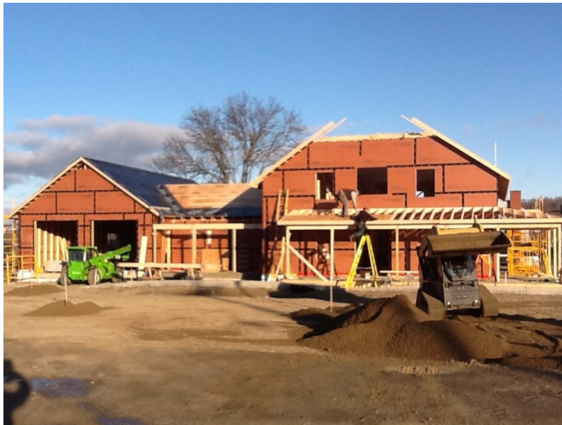
Construction Progress on New Police Station as of 10/29/13
