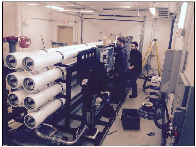
The ISI Nanofiltration system skid is in place in the new Water Treatment Facility and being interconnected with the other systems.
